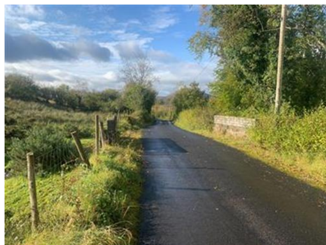
Figure 26 - Bridge 11 within L-6180
