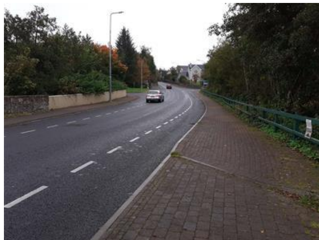
Figure 24 - Bridge 9 within R-282
