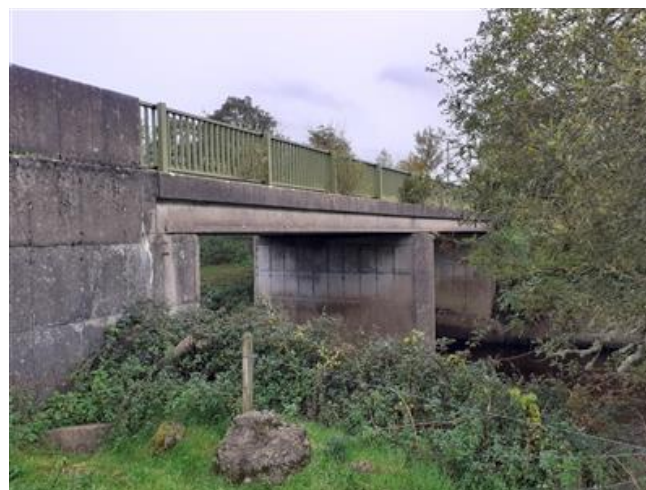
Figure 18 - Bridge 3 within L-4165
