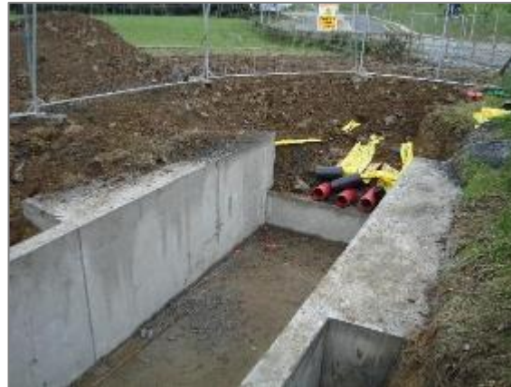
Figure 9 - Completed joint bay prior to cable installation (in-situ)
