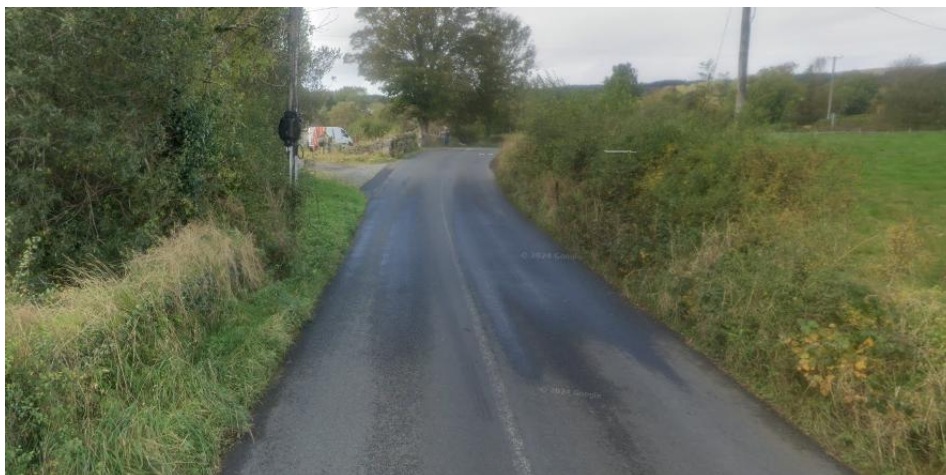
Figure 20 - Bridge 5 within L-4166
