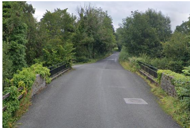
Figure 23 - Bridge 8 within L-22136
