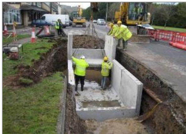
Figure 10 - Typical joint bay under construction (pre-cast)
