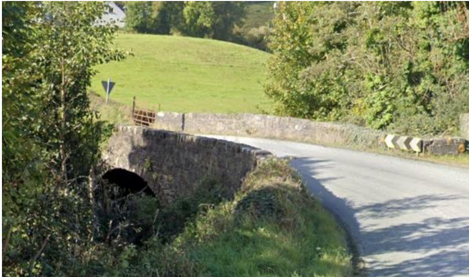
Figure 17 - Bridge 2 within L-4263
