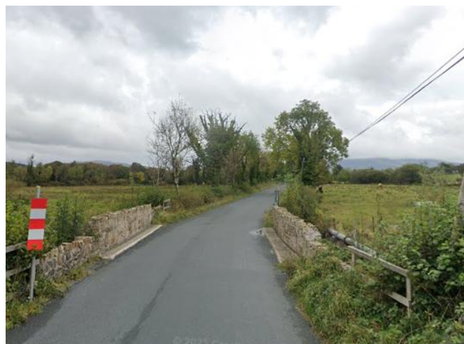
Figure 22 - Bridge 7 within L-2169
