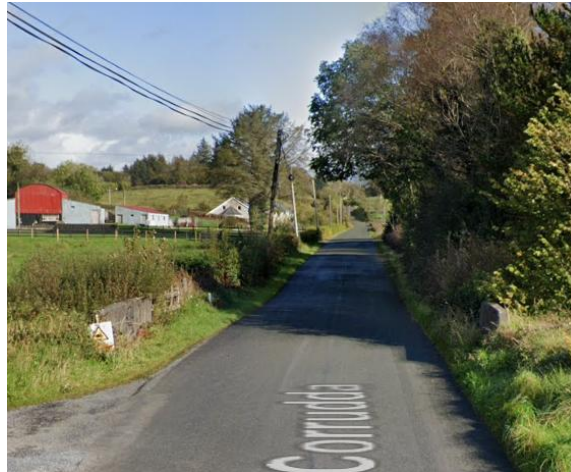
Figure 19 - Bridge 4 within L-4166
