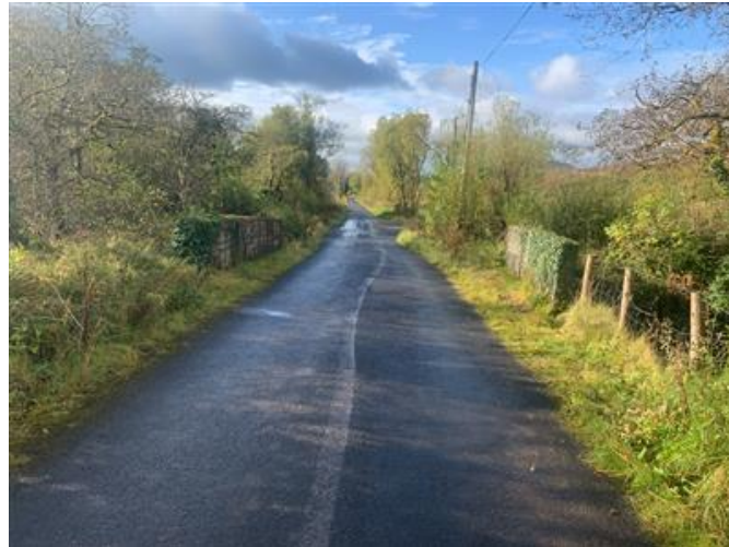
Figure 25 - Bridge 10 within L-6180
