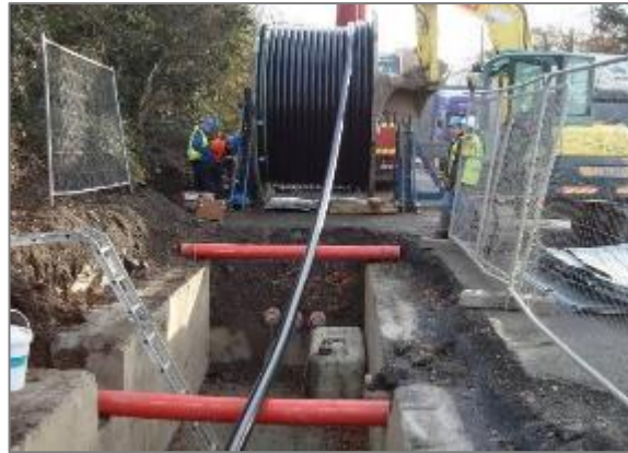
Figure 11 - HV cable pulling procedure (Typical drum set-up)
