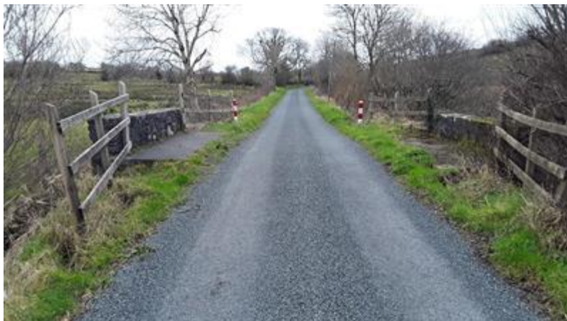
Figure 16 - Bridge 1 within L-5204
