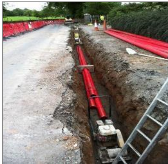
Figure 3 - Typical 110kV Underground Duct Installation
