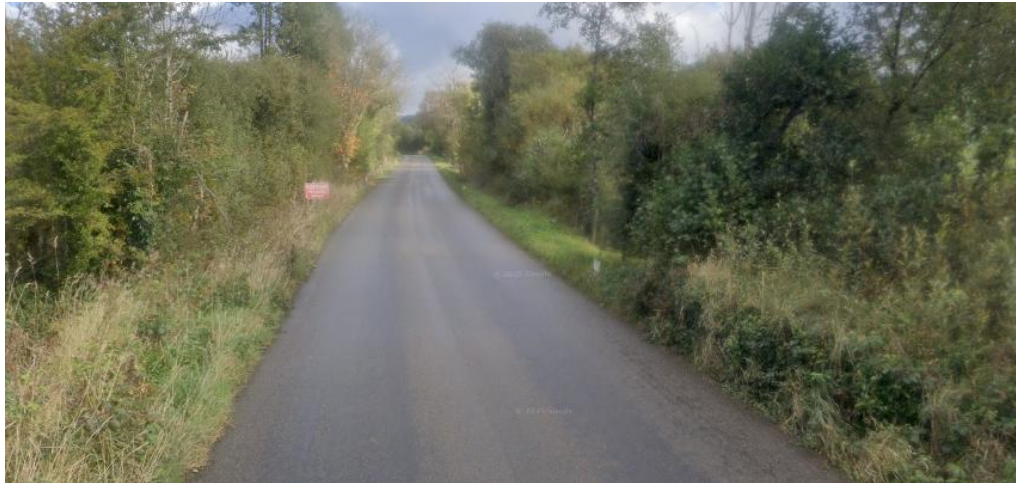
Figure 21 - Bridge 6 within L-2169
