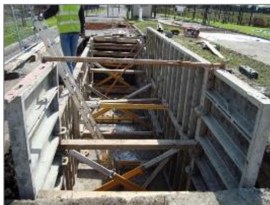
Figure 8- Typical joint bay under construction (in-situ)
